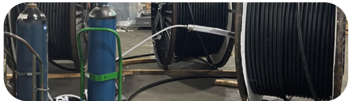
Purging cables using compressed nitrogen gas.
