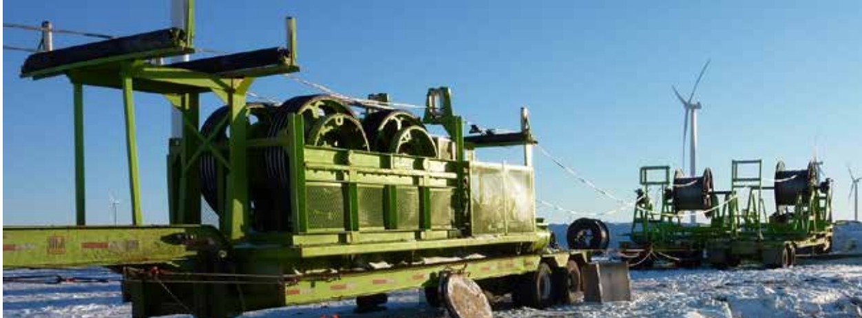
Figure 4. Payoff and bullwheel setup.
